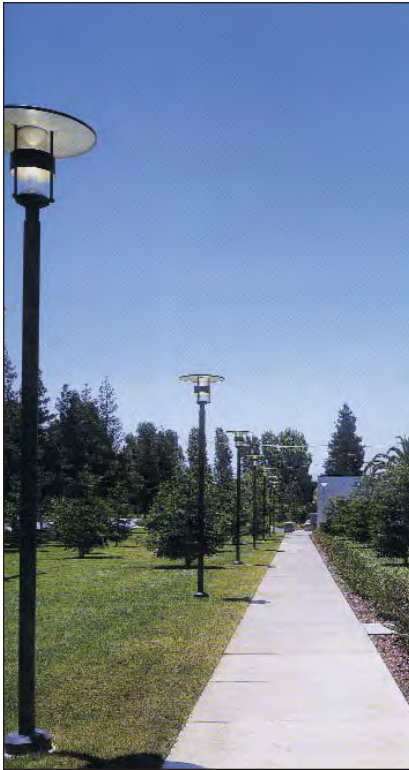
Shielded, largely indirect pedestrian light. High pressure sodium lamp, aluminum base and pole. (Louis Poulsen Lighting, Inc. Photo by Frank Domin Photography)
